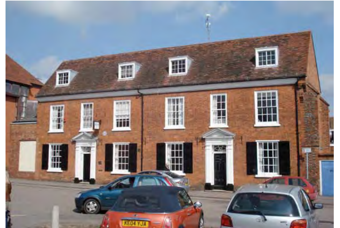
View from Portmill Lane car park of the Listed Building at No.7 & 8 Portmill Lane
