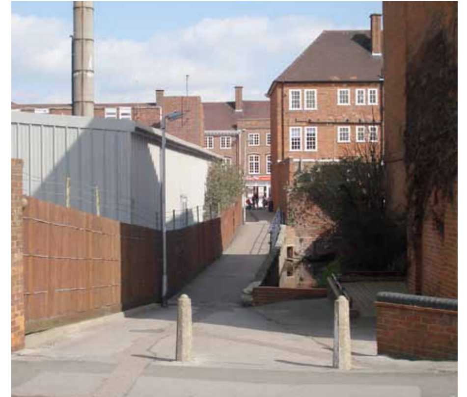
View of existing River Hiz walkway
