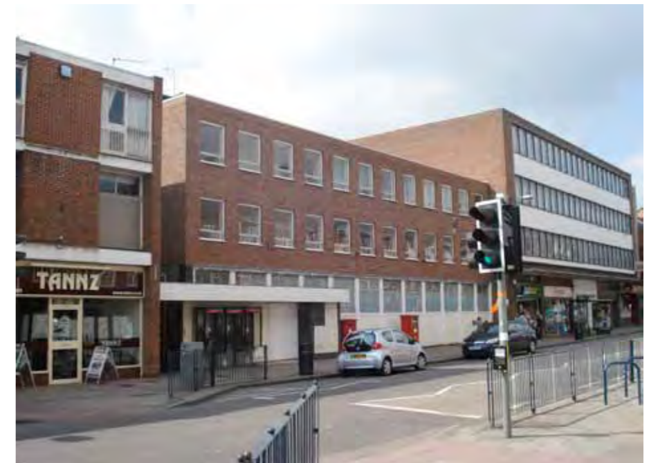
View of the Royal Mail Delivery Office in its context along Hermitage Road
